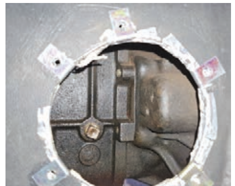
...giving good access to the filler plug when the plate was removed.
